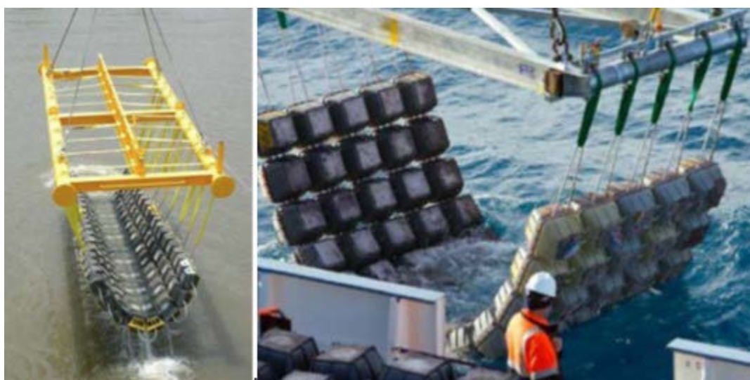
Figure 4-15 Concrete mattress deployment (courtesy of FoundOcean)
