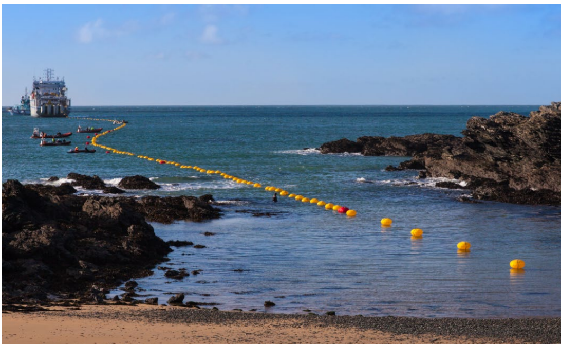
Figure 4-20 Example of a cable being floated-in
