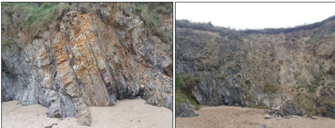
Figure 6-3 Cliffs at Baginbun Beach (left image showing close-up of rock strata)
